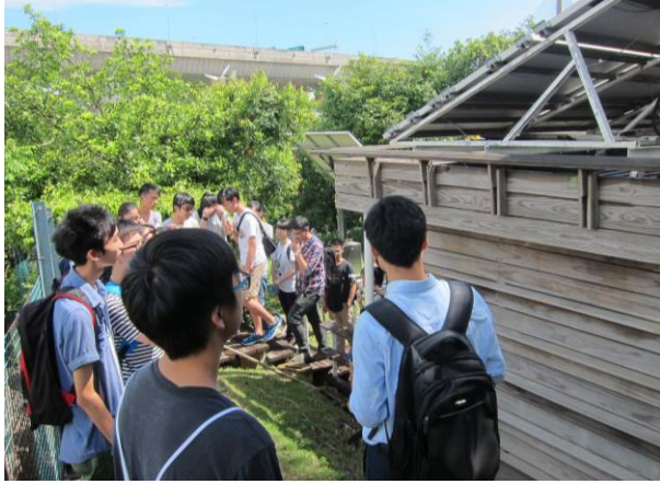
Rooftop Solar PV Shelter
