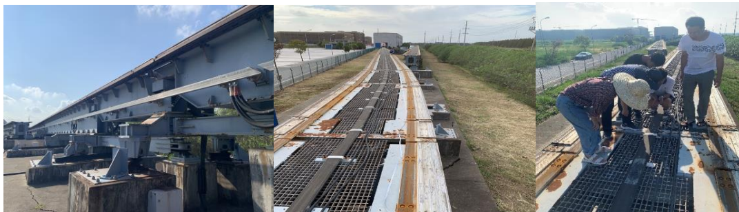
Figure 2. 5 Turnout of mid-to-low speed maglev rail line
