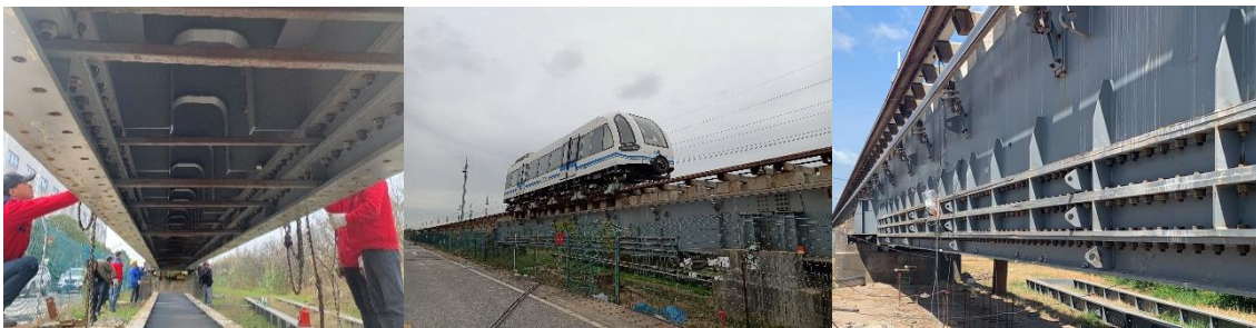
Figure 2. 3 Steel box-girder with adjustable height
