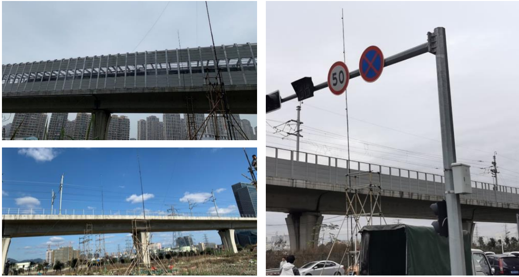
Figure 2. 11 Noise and vibration test of Wenzhou S1 line in January 2020
