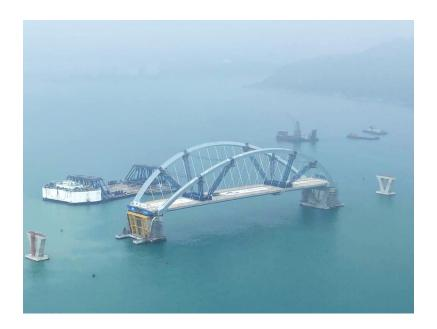
A total of 4,400 tons S690 steel plates were adopted to make the two curved box sections, and their cross-sectional dimensions vary from  $3.0 \times 3.0 \times 3.5 \times 3.5 \text{ m}$ .
