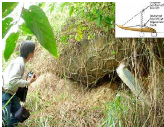
Barrier holding back much of the debris
