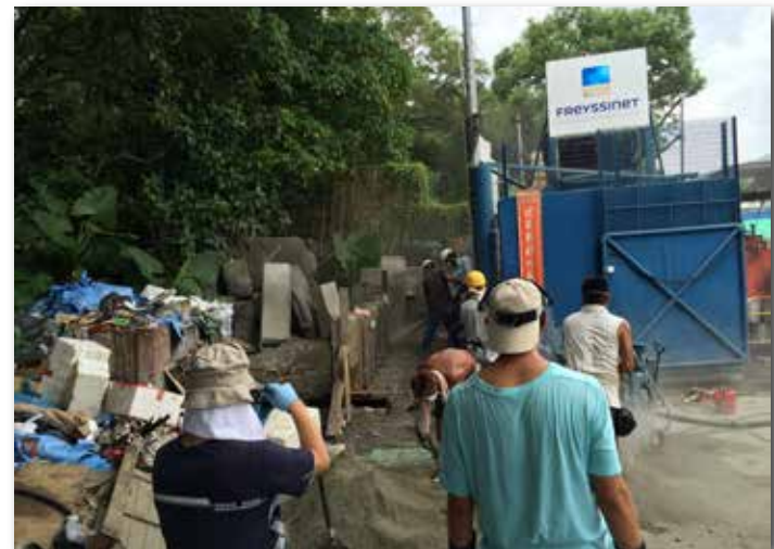
Application of dry spray shotcrete (jointly with Freyssinet)
