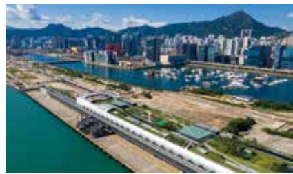
Land Reclamation 填海
