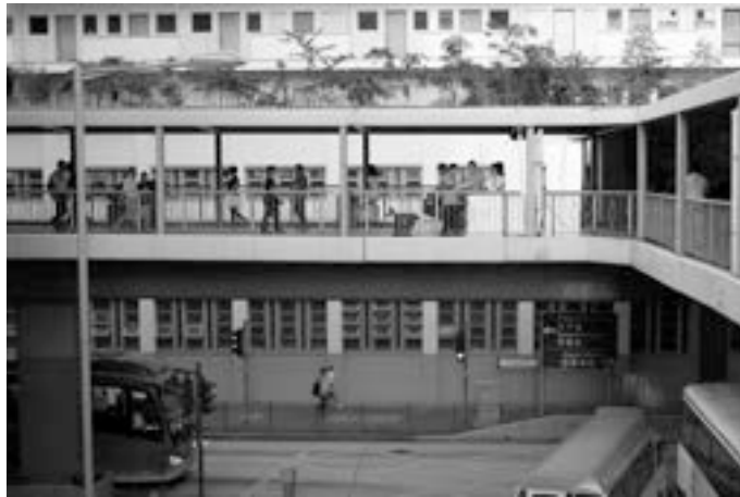
Figure 5-25 To improve the urban traffic efficiency in densely populated urban areas, pedestrian bridges are used to segregate pedestrian and vehicular traffic; pedestrians are isolated between the ground and elevated levels.
