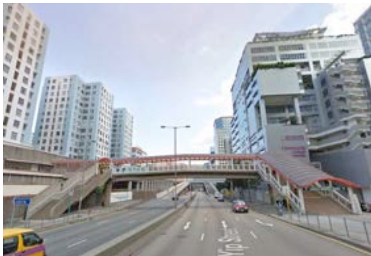
Figure 4-9 Pedestrian bridge at 33 Wai Yip Street, Hong Kong (Source: Google Maps)
