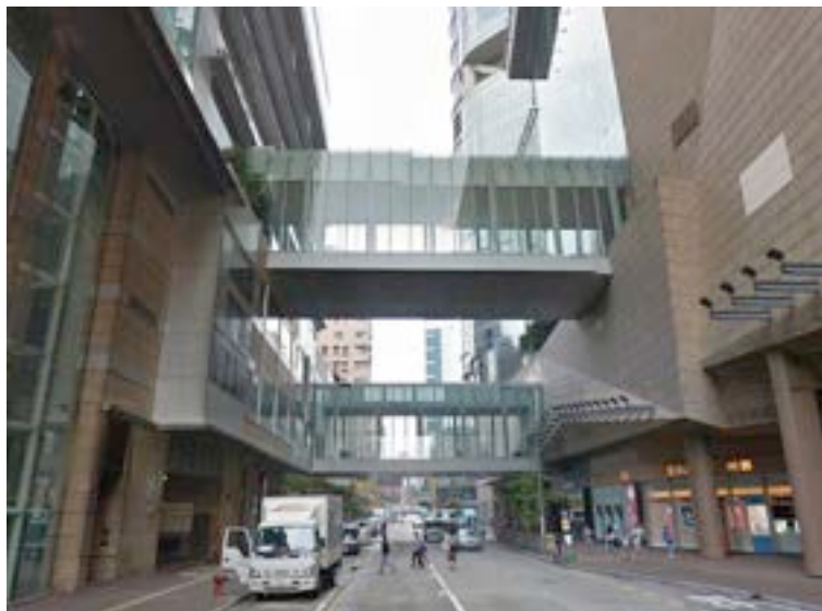
Figure 4-13 Pedestrian bridge over Langham Place (Source: Google Maps)
