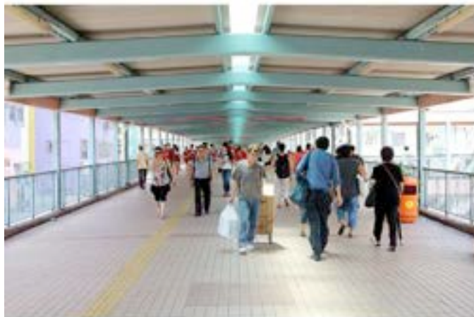
"Necessary activities-dominant" bridge use pattern
