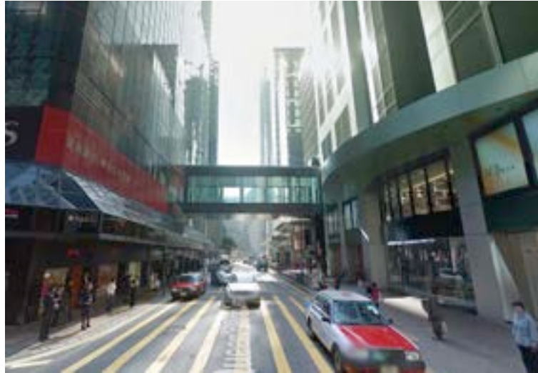
Figure 4-10 Pedestrian bridge at 28 Queen's Road Central, Hong Kong (Source: Google Maps)
