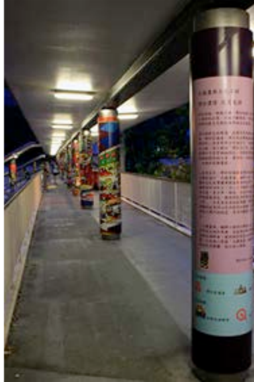
Figure 4-22 Wan Chai footbridge gallery
