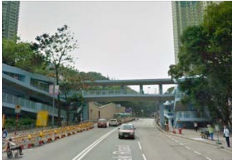
Figure 4-8 Pedestrian bridge at 111 Fung Tak Road, Hong Kong (Source: Google Maps)
